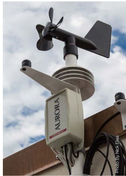
Redwood Electric Group wired the weather station on top of the facility.
