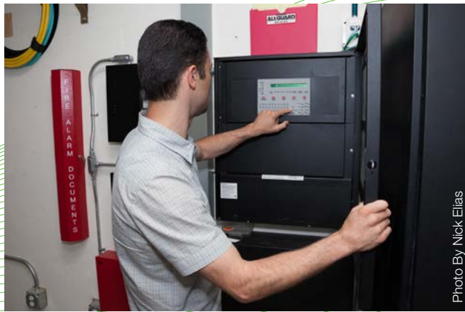
Redwood Electric Group installed a Notifier fire alarm system.
