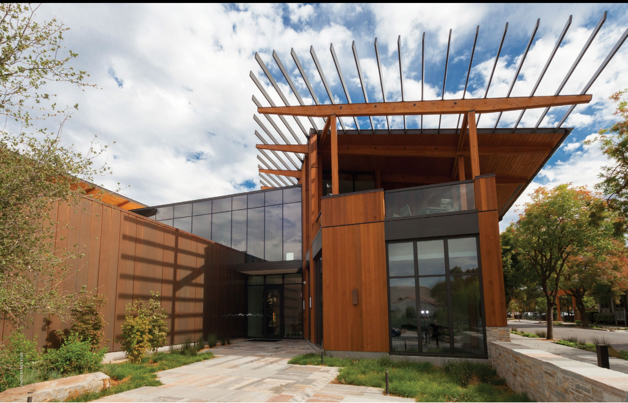
The David and Lucile Packard Foundation's offices have obtained LEED Platinum Certification and have been designed as a NetZero Energy facility.
