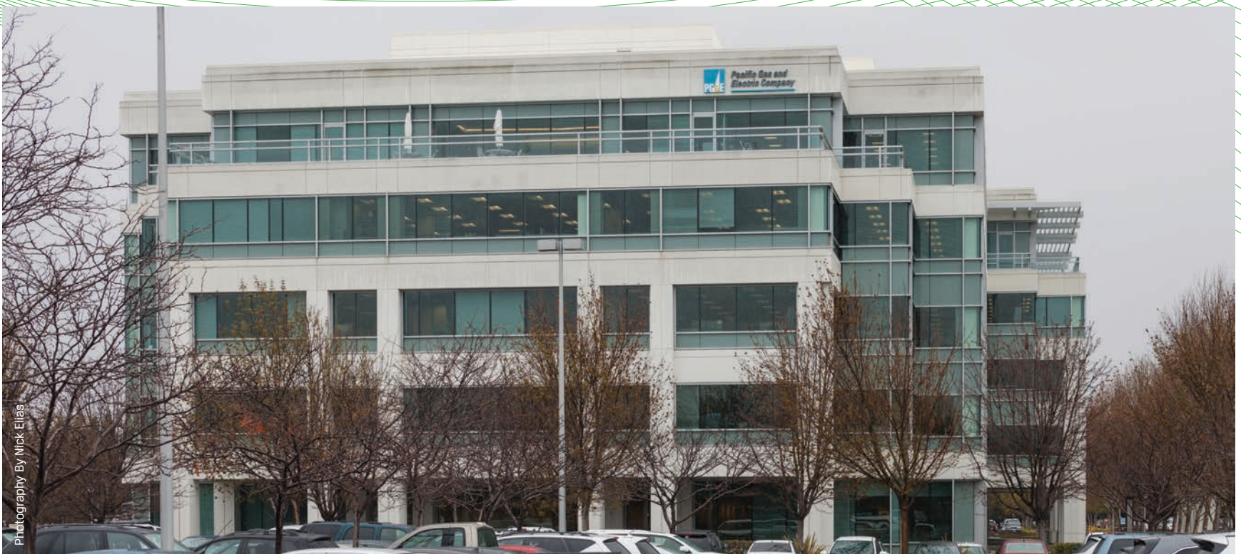
CH Reynolds wired the on-site data centers at PG&E's new Gas Operations Center with over 100 miles of network cables.
