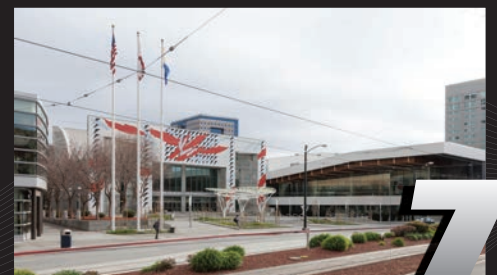
Redwood Electric Group Wires New San Jose Convention Center.
