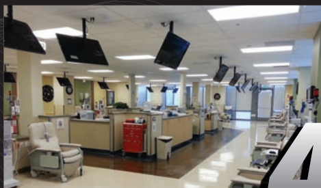
Silver Creek Electric Wires New State-Of-The-Art Dialysis Center in San Francisco.
