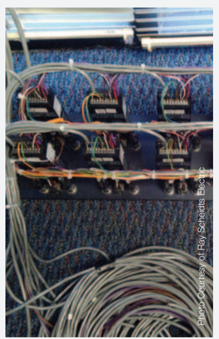
Image of the back of the Variac heat flux control panels built and installed by Ray Scheidts Electric.
