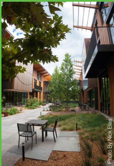
The David And Lucile Packard Foundation recycled many of the materials from its old site before building its new headquarters.
