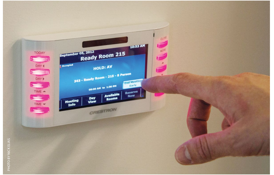
Redwood Electric Group wired control panels outside each conference room to allow Foundation staff to reserve meeting time.
