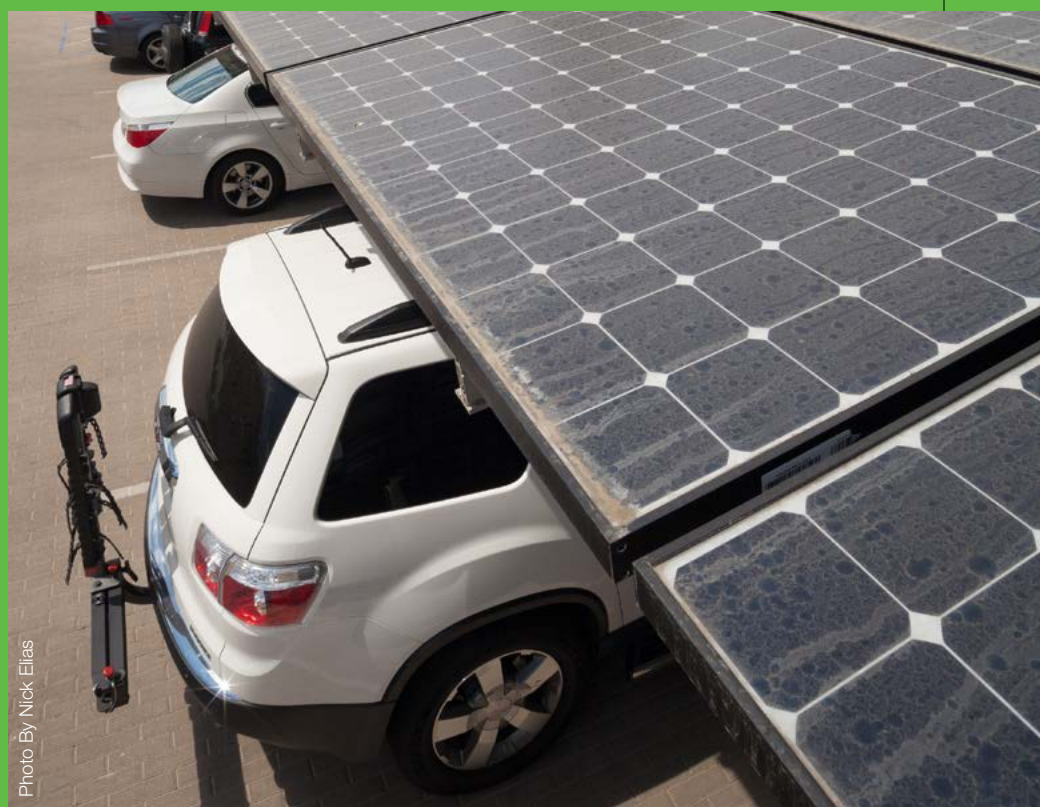
Redwood Electric Group installed part of the photoelectric system on the roof of the parking garage.
