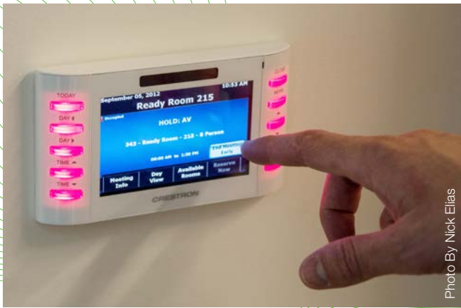
Redwood Electric Group wired control panels outside each conference room to allow Foundation staff to reserve meeting time.
